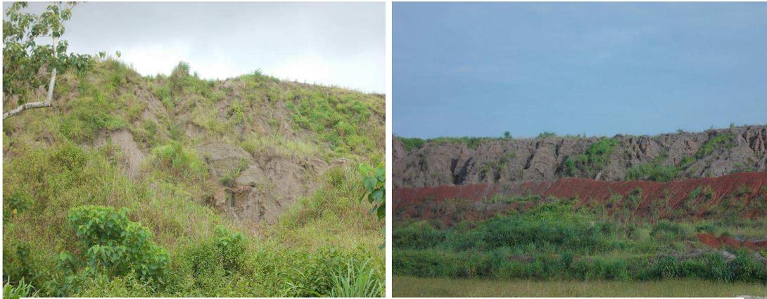
**Figure 12 - Huge dumps of inert tailings dumped at the iron ore mines in Lunsar after the extraction of the ore.**
